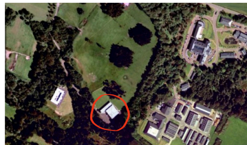
EPCC Advanced Computing Facility, 2014
