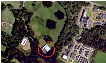
EPCC Advanced Computing Facility, 2014
